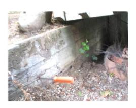
The post and rails of the 3 Eastern retaining walls are significantly rotted and are considered to have lost all structural integrity and should be replaced immediately.
