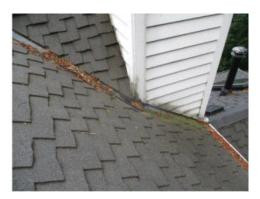
There is fortiflash exposed under the livingroom door. This material is not UV rated and should be covered.
