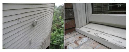
The bottom edges of the siding are not completely painted or sealed. This is an important area to have properly painted or sealed to prevent water damage, paint lifting, and peeling.
