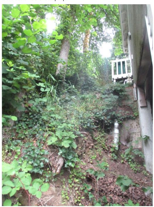
There is a large portion of the Western slope that is over a 45 degree slope, has multiple tall trees, was excavated, and is unsupported.
