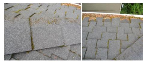
There is a build up of moss on the roof that should be cleaned and/or treated to facilitate the expected life of roofing.
