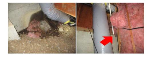
There are water stains or signs of active leaking into the crawlspace all along the area of the driveway attachment to the house and where the concrete driveway was poured over the siding on the side of the house. There is no current elevated moisture readings at the water stains in these areas; however, it does appear that leaking has been seasonal and reoccuring.
