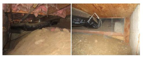
There is restricted clearance in the crawlspace and the flooring insulation is hanging and damaged. These two issues combined are significantly restricting both visual and physical access throughout the crawlspace. A reasonable attempt to inspect the crawlspace was made however; hidden or unapparent issues may exist due to the limited access.
