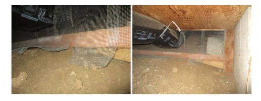
INSULATION & DUCTING There are areas where the floor insulation has been knocked or pulled down from the supports. It would be recommended to re-install and to secure these areas. There is no twine or batten to hold or support the flooring insulation. The insulation should be
